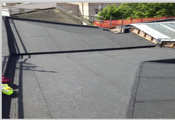
Photo 2 Completed roof section.
