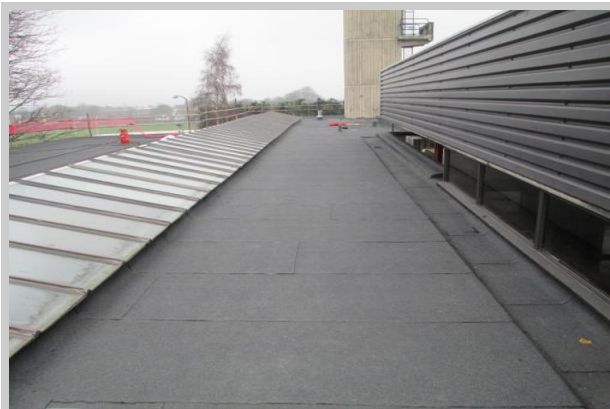
Completed flat area with internal gutter detail.
