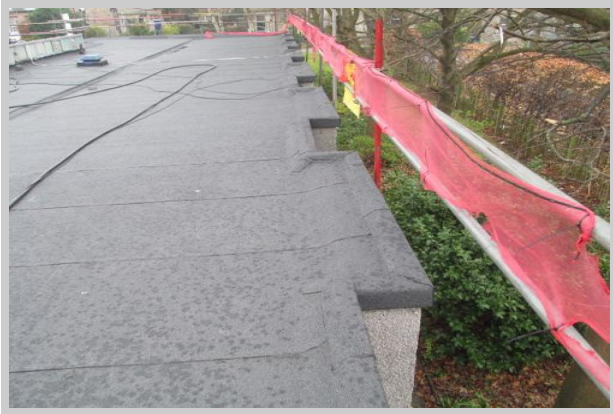
Welting drip detail completed to perimeter edge.
