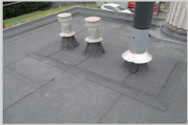
Neat and tidy detailing work to vent pipes.
