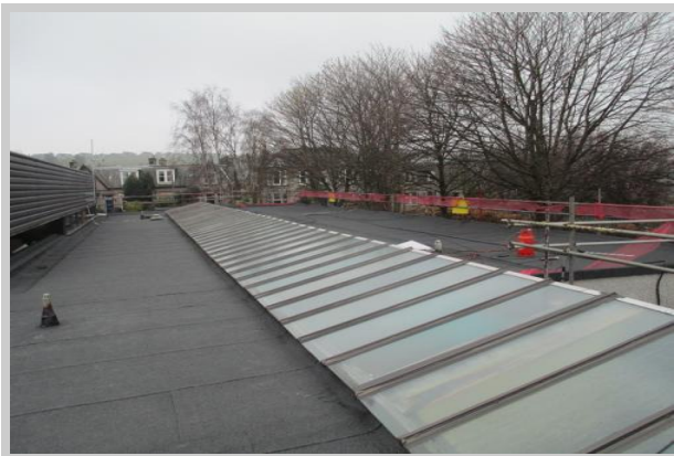
Overview of completed works.
