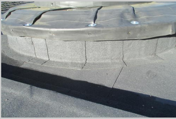
Detailing work completed to roofline on the high level roof.
