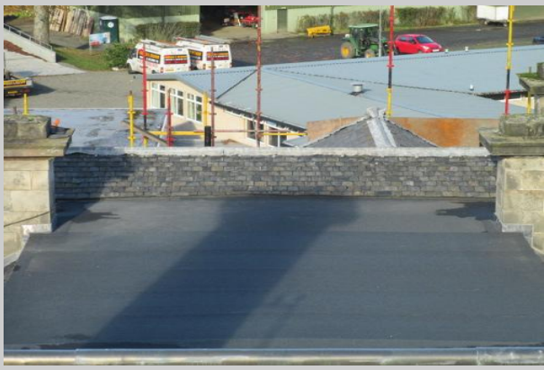
Overview of low level roof.
