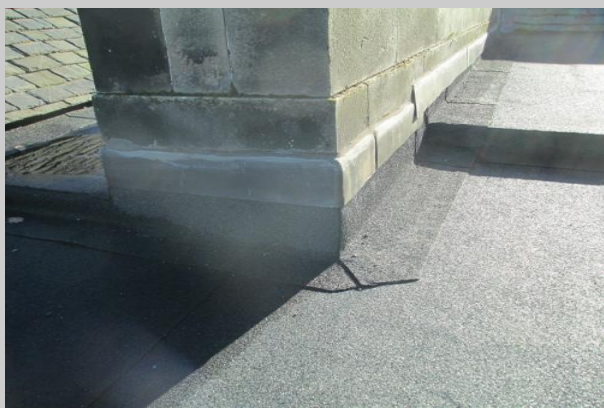
Completed detailing work to high level roof.
