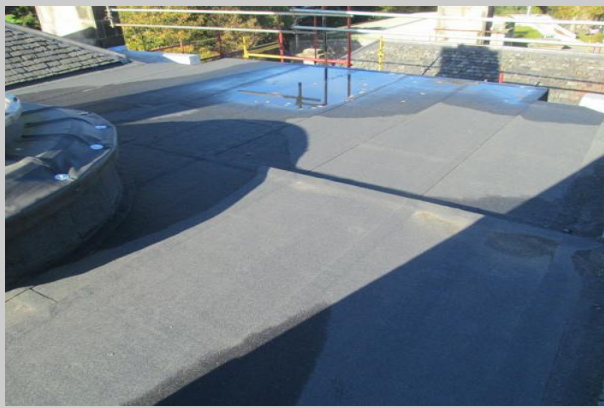
Overview of completed high level roof.
