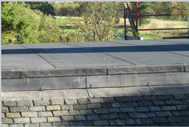
Low level roof showing welted drip detail.
