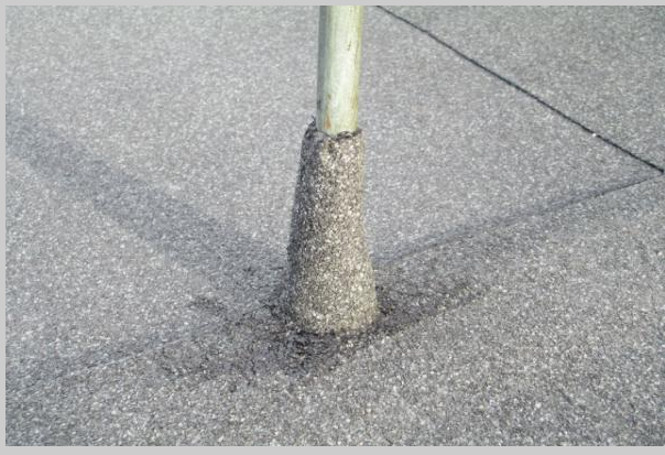
Neat collar detail round pipe outlet.
